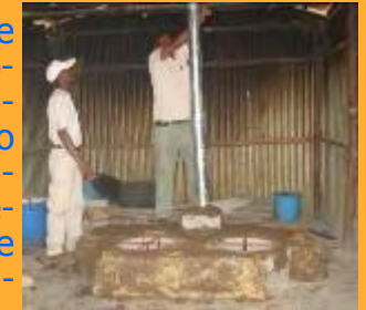
Mirt stove being installed
